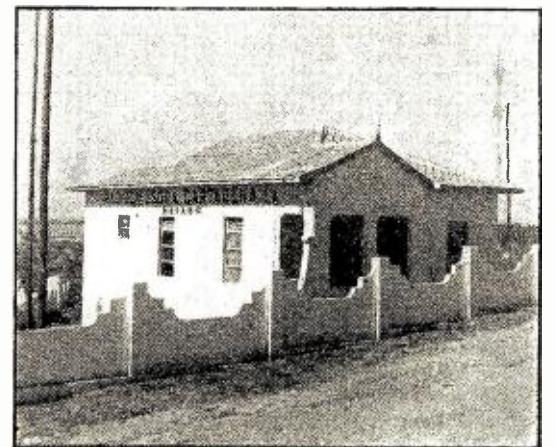
A "VERI" AND ITS STATION Observer J. S. Chokan, Jr., of Cleveland, Ohio, received the above card from HJ1AP. The transmitter house is also pictured.
